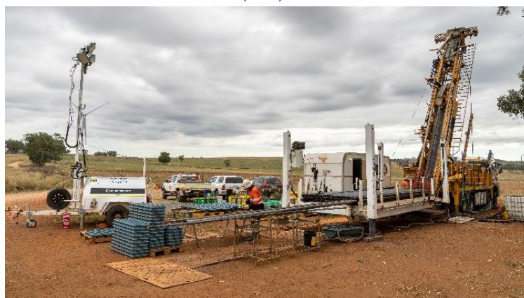
Diamond drilling uses similar equipment to a water bore.
