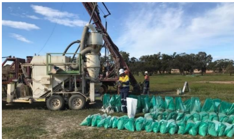
Air Drilling may use a truck-mounted rig to collect rock chips and be completed quickly.
