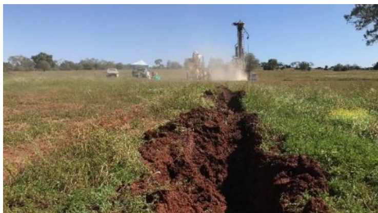
Costeaning or trenching allows a geologist to collect sub-surface samples.
